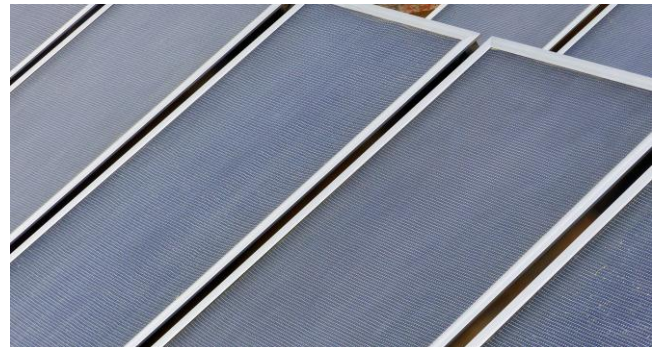
Picture 1: Honeycomb collectors at Urim.
