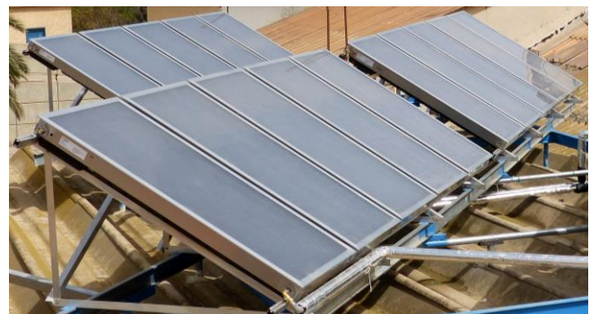
Picture 2: On the roof of the laundry
